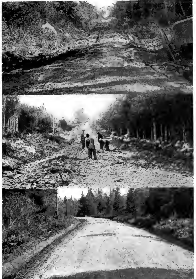
Good Roads in Compton, P.Q., Macadam built in 1915, Road before, during and after construction.
